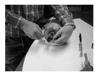
Install SAE pump mount to motor C-face, align bolt holes.
